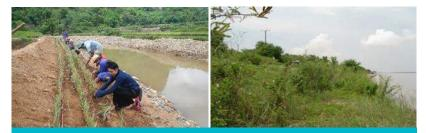
**Riverbank stabilization.** Vetiver grass planted along a riverside in northern Viet Nam (left) and the grassed flood foreshore with small trees on an embankment in Cambodia (right) provide for riverbank stabilization (photos by the International Centre for Environmental Management and J. Howell).
